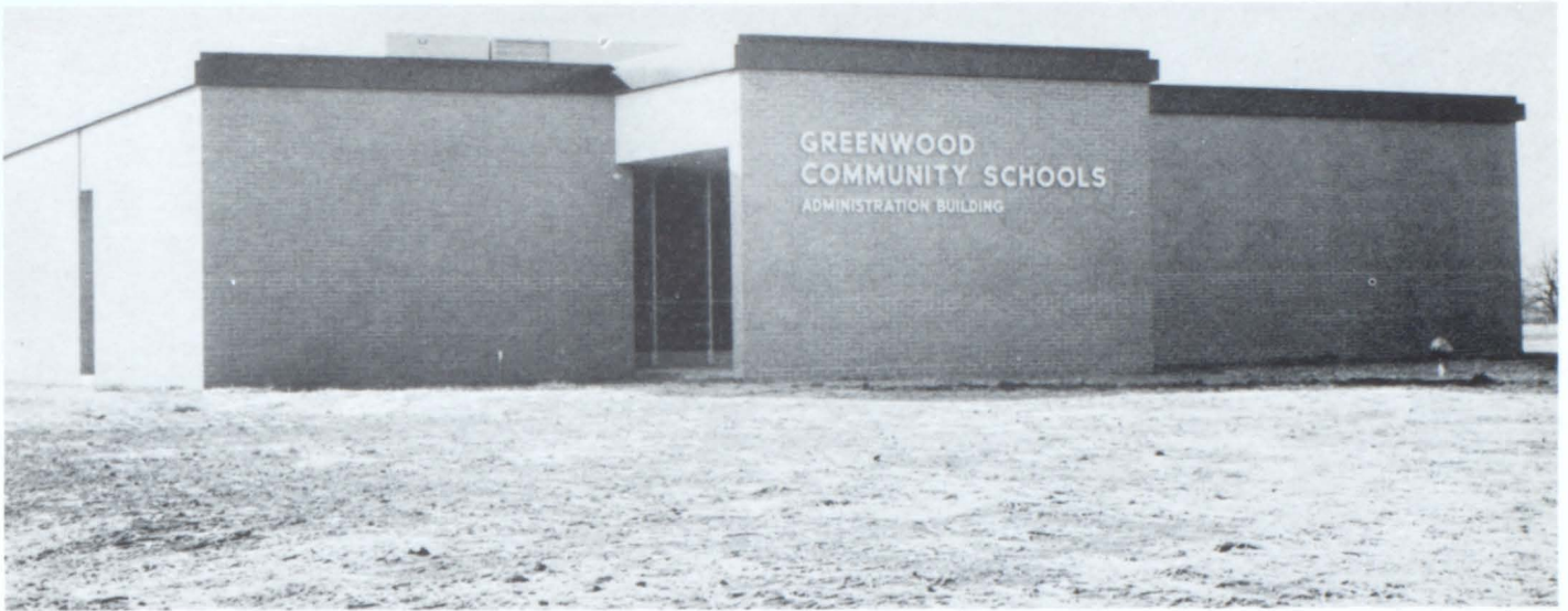
The new Greenwood Community Schools Administration Building was located on Smith Valley Road.
